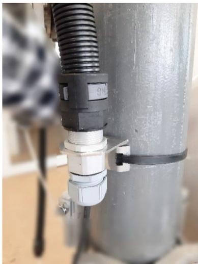
**7** Fasten another end of fiber conduit to the pole using included tie-wrap.
