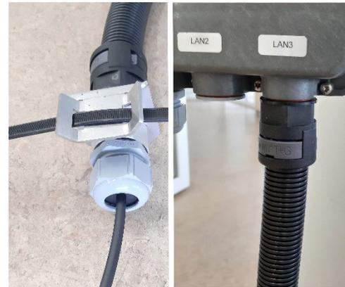
**6** Tighten parts on both ends of the conduit to weatherproof assembly. Do not break the cable.
