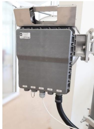
**8** Assembled view of the Integra-E/E2/E3 with optical cable conduit. Cables must always be at the bottom of the Integra-E/E2/E3.
